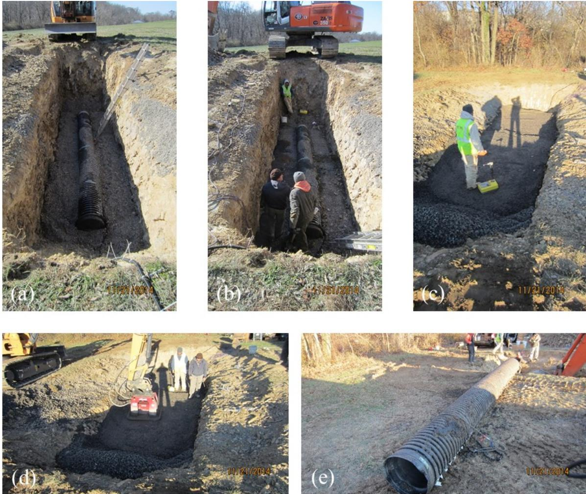
**Figure 4.36 Photos showing various stages of field test: a) pipe in trench; b) placement of pressure cells on side along mid elevation of pipe; c) nuclear density gauge testing; d) compaction using a hydraulic plate compactor; e) retrieved pipe after test**
