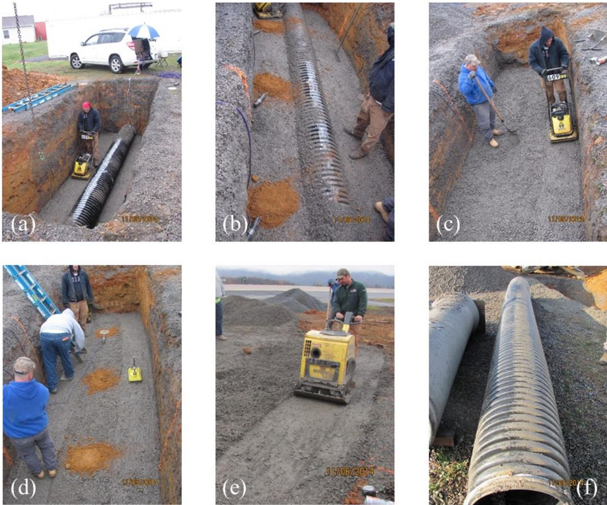
**Figure 3.20 Photos showing various stages of field test: a) compaction using a small tamper on side of pipe; b) placement of pressure cells on side along mid elevation of pipe; c) compaction using a small tamper on top of backfill zone; d) placement of pressure cells on top of pipe and nuclear density gauge testing; e) compaction using a walk-behind vibratory roller compactor after last lift; f) retrieved pipe after test**
