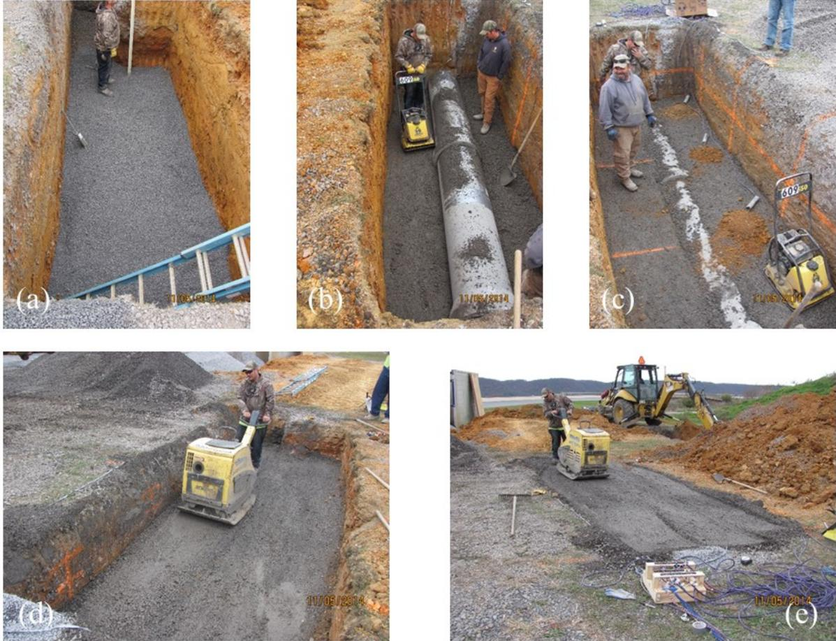
**Figure 3.15** Photos showing various stages of field test: a) measuring AASHTO #8 bedding; b) compaction using a small tamper on side of pipe; c) placement of pressure cells on side along top of pipe; d) compaction using a walk-behind vibratory roller compactor in cover zone; e) compaction after last lift and data acquisition system with wires
