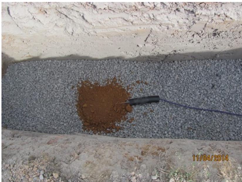
**Figure 3.4** A photo showing placement of a pressure cell 6 inches above pipe
